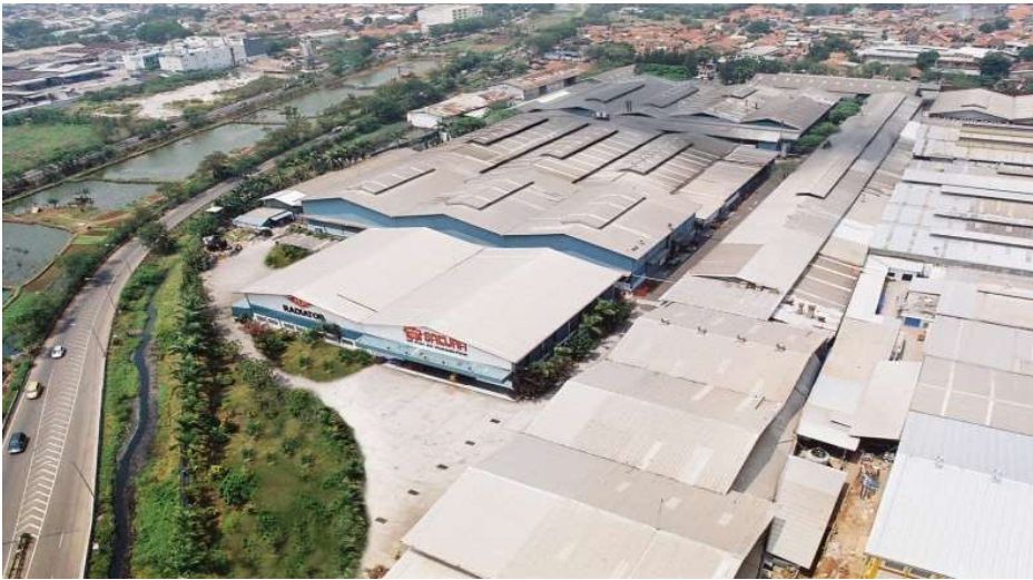
Kapuk Plant (Radiator Facilities)
